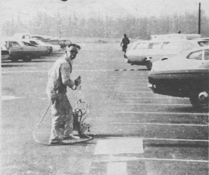
Bob Plumlee, a LBCC custodial engineer, finishes painting signs on Handicapped parking stalls on the south parking lot. He casts suspicious glances at on-the-spot photographer, Bob Byington.
