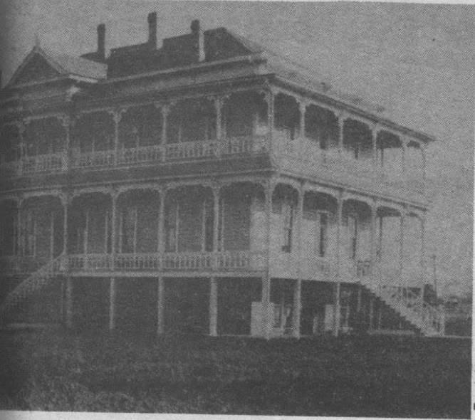
as a girl's dorm as well as classrooms. The name in three mountains or "Three Sisters." The building still the present Bureau of Mines site.
