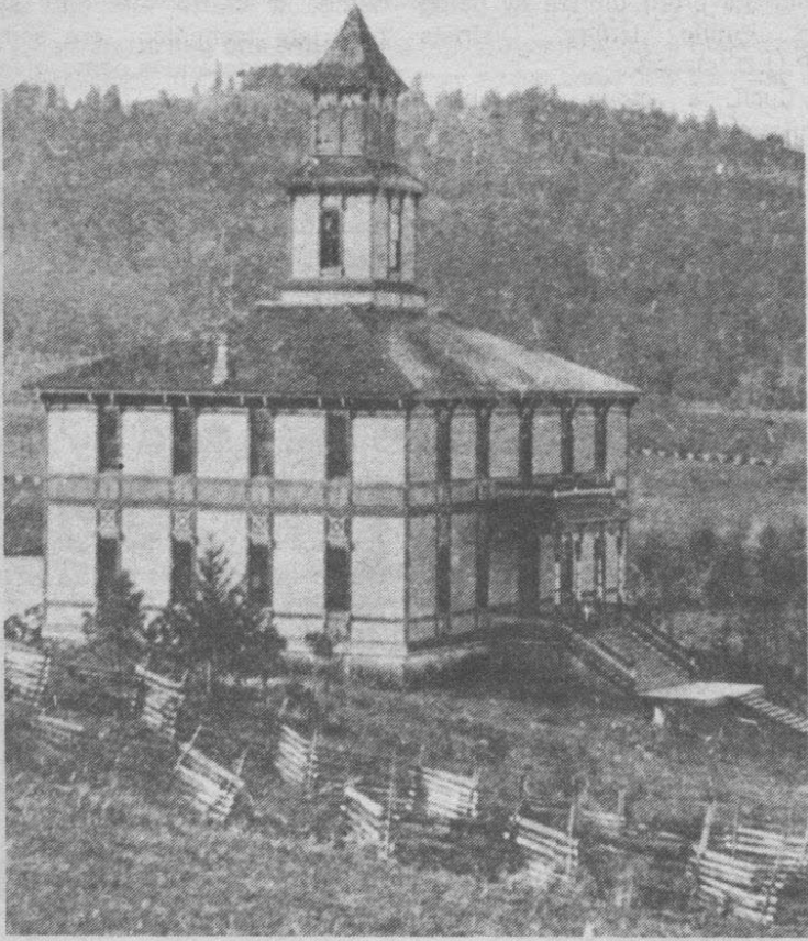
THE OLD MINERAL SPRINGS COLLEGE building was one of a variety of major landmarks during Sodaville's heyday in the 1890's.
