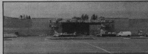
Work continues on the new Wal-Mart store under construction in Lebanon.
