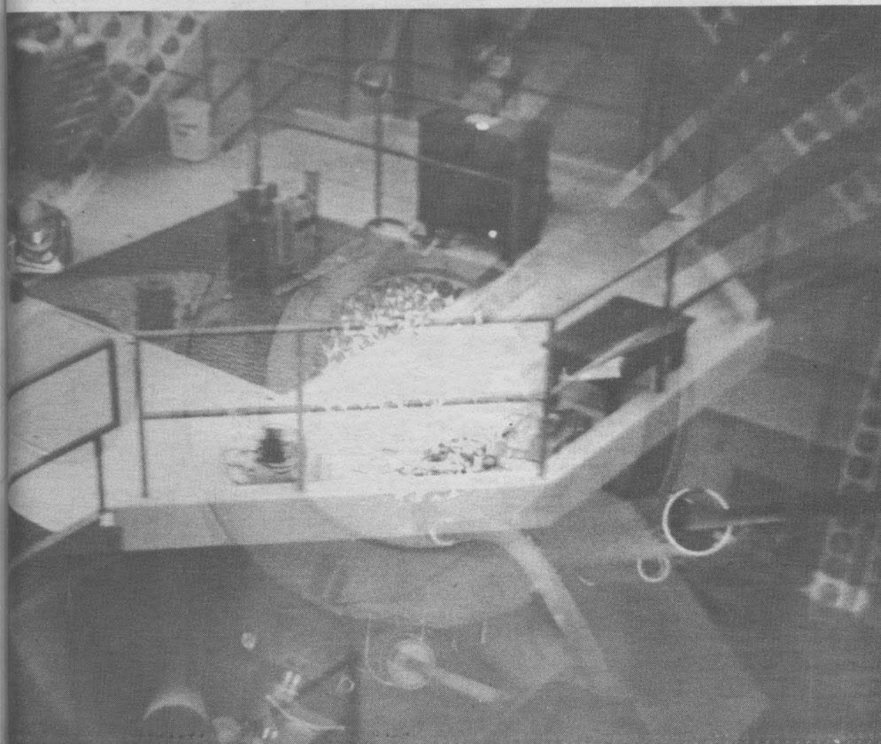
A special-effect double exposure shows the core of the reactor through 16 feet of water superimposed on the reactor itself. The view of the core was taken through the square grid on top of the reactor.
