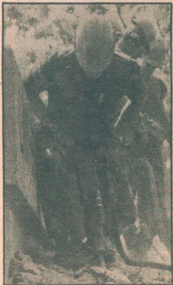
A guardsman uses a jackhammer to chisel away concrete.
